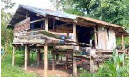
Figure 3: Typical of poorly constructed wooden + corrugated zinc house.
