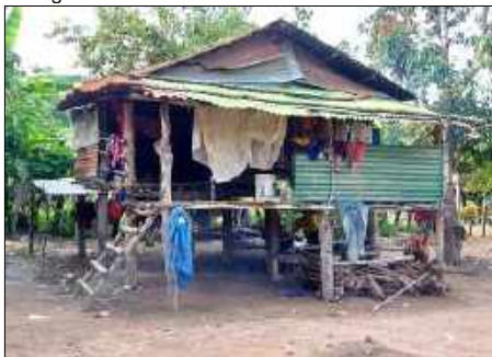
Figure 2: Typical of poorly constructed wooden + corrugated zinc house.
