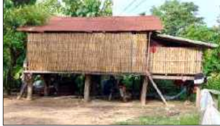
Figure 4: Typical of poorly constructed bamboo + corrugated zinc house.
